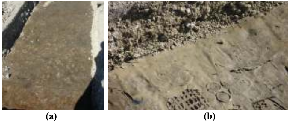
Figure 4.31. Section 13BW subgrade a) after the geotextile removed and b) the zoomed in view after geotextile removal.
