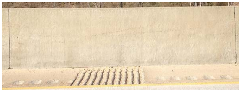
Fig. 3.1-1 Barrier wall section minimal deterioration, (e.g. no visible map cracking).
