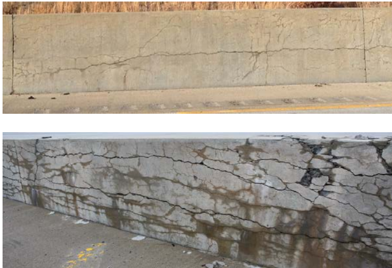
Fig. 3.1-2 Barrier wall section moderate deterioration, (e.g. moderate visible map cracking, and a longitudinal crack along the full length of the section) (Top). Barrier wall section severe deterioration, (e.g. severe map cracking, longitudinal cracks, crushing at the joints, and visible alkali-silica gel exudation) (Bottom).
