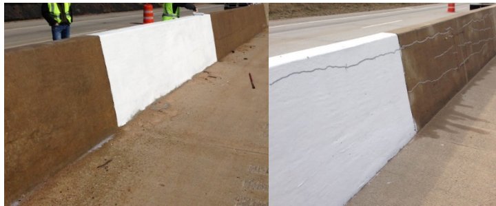
Fig. 3.3-4 Application of surface treatment (left) and crack sealant (right).
