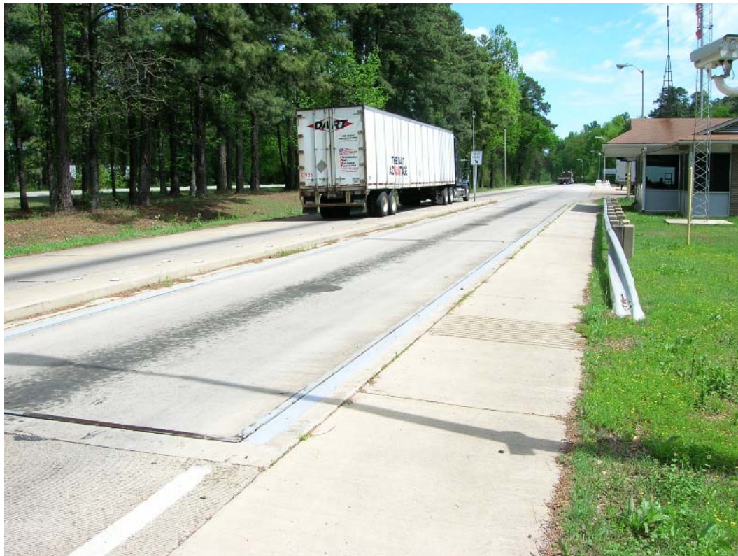
Figure 3-3: Hope Weigh Station Building and Static Scales
