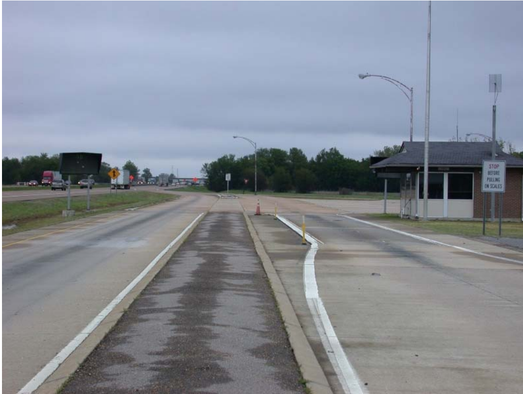
Figure 3-7: Lehi Weigh Station Building and Static Scales
