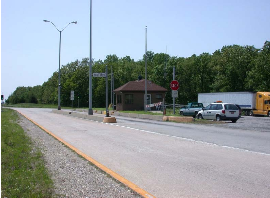
Figure 3-5: Joplin Weigh Station Building and Static Scales
