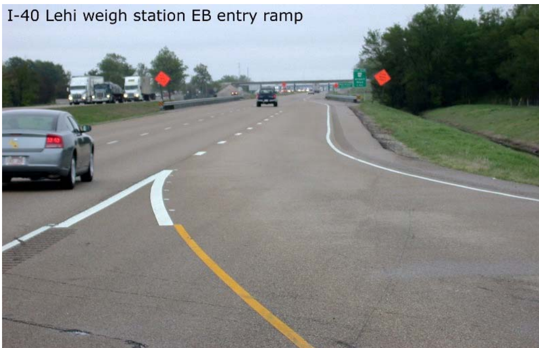
Figure 3-8: Lehi Weigh Station Freeway Acceleration Lane
