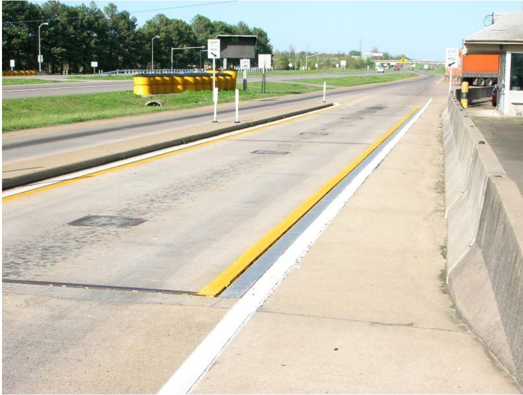
Figure 3-1: Alma Weigh Station Building and Static Scales
