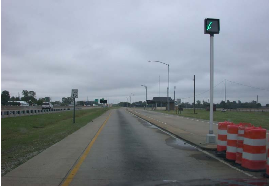
Figure 3-9: Marion Weigh Station Building and Static Scales
