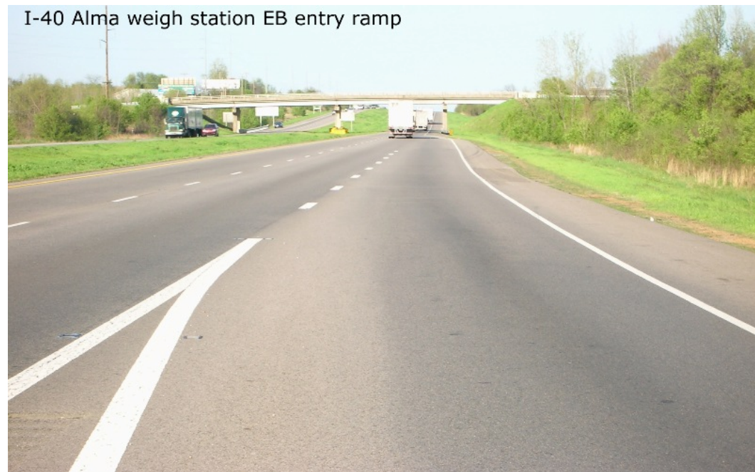
Figure 3-2: Alma Weigh Station Freeway Acceleration Lane
