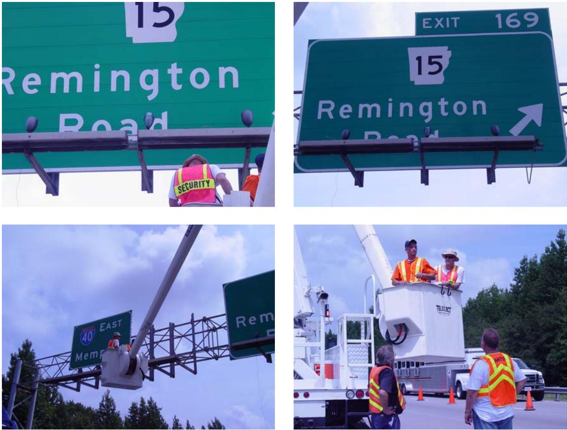
Fig.27 Installation of New CFL Light Fixtures
