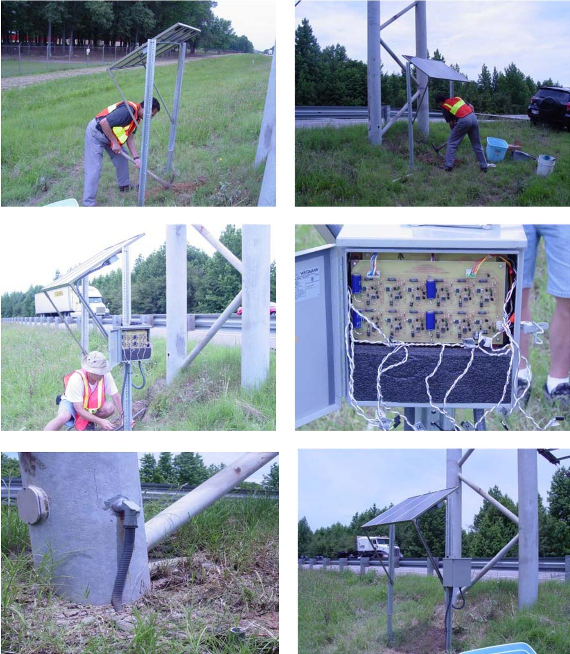
Fig.24 Installation of CFL Control Box (Late June 2007)
