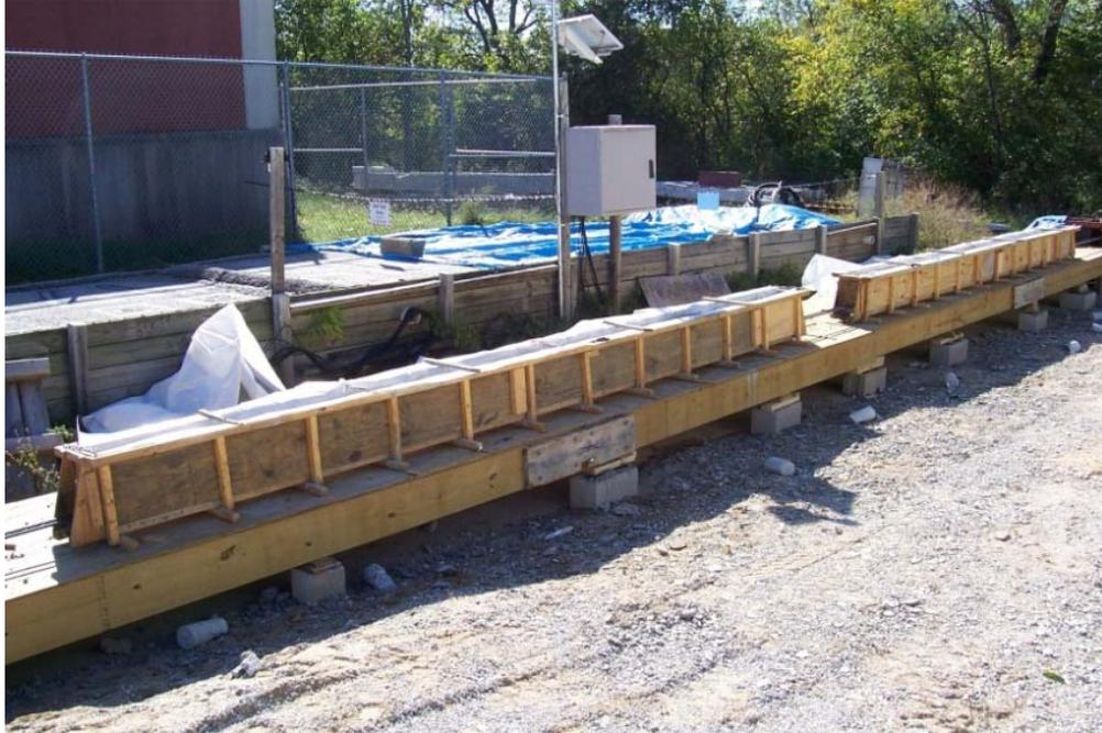
**Figure 3.6 Beam Formwork**
