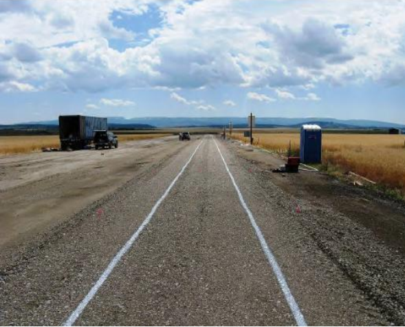
Figure 2.5: Full-scale field testing (Cuelho and Perkins 2009).
