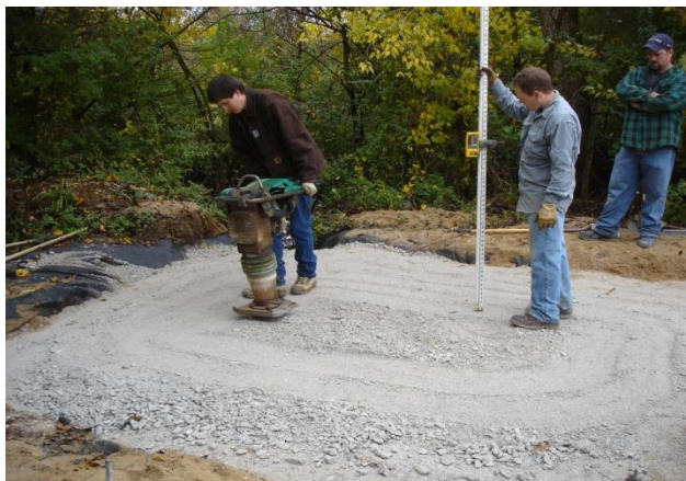
Figure 4.5: Compacting Class 7 base course layer with the whacker packer.
