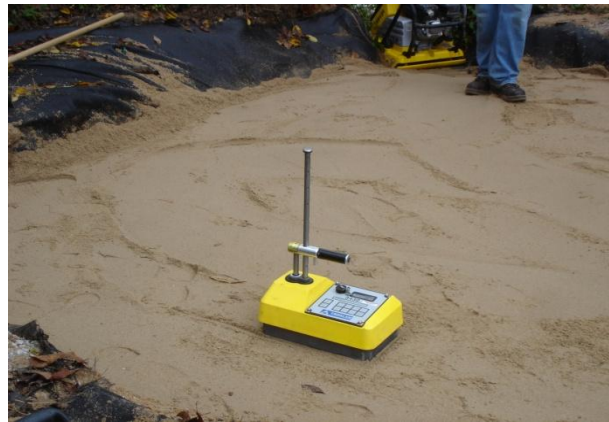
Figure 4.4: Nuclear density reading on the sand layer.
