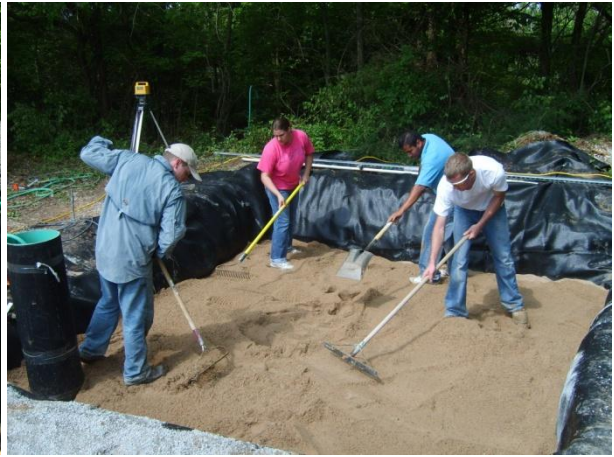
Figure 3.10: Placement of 6'' sand layer.
