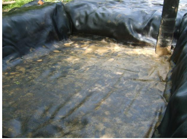
Figure 3.8: Geotextile lined test pit.
