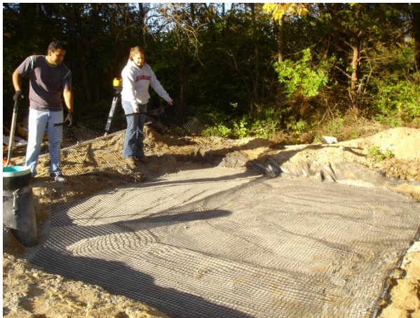
Figure 4.9: Placement of the geogrid in the test section.
