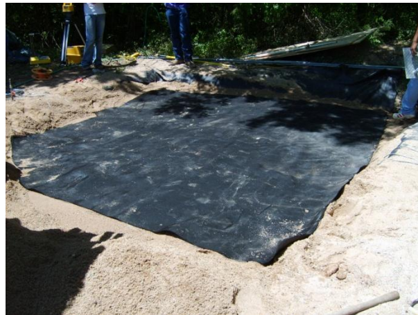
Figure 3.18: Geotextile placement.
