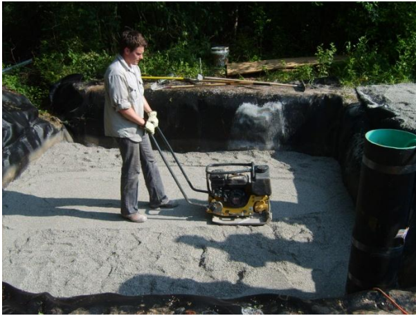
Figure 3.9: Compaction of 8'' gravel layer.
