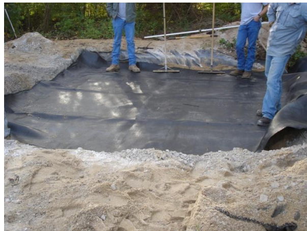
Figure 4.10: Placement of the geotextile in the test section.
