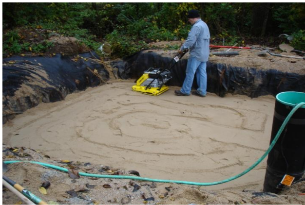
Figure 4.3: Compacting 6" sand lifts with the vibratory plate compactor.
