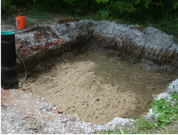
Figure 3.7: Construction of the test pit.
