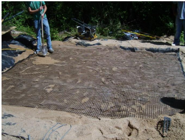
Figure 3.17: Geogrid placement.
