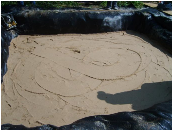
Figure 3.11: Compacted sand layer.
