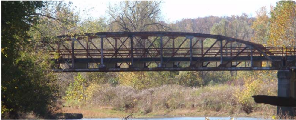
FIGURE 1 Elevation view and photograph of typical Parker pony truss span.
