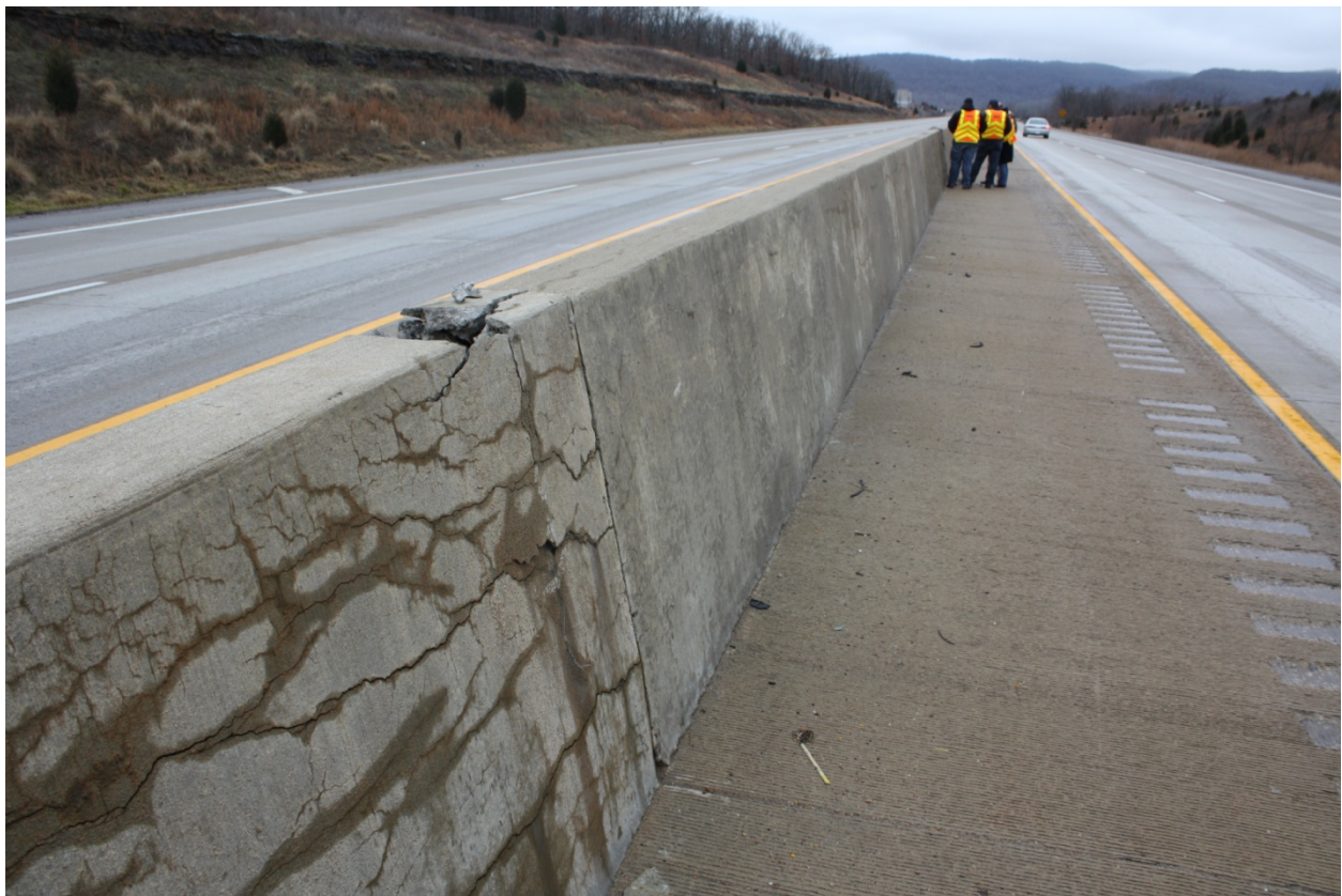
Figure 1. Good and Poor Sections of the I-540 Wall.
