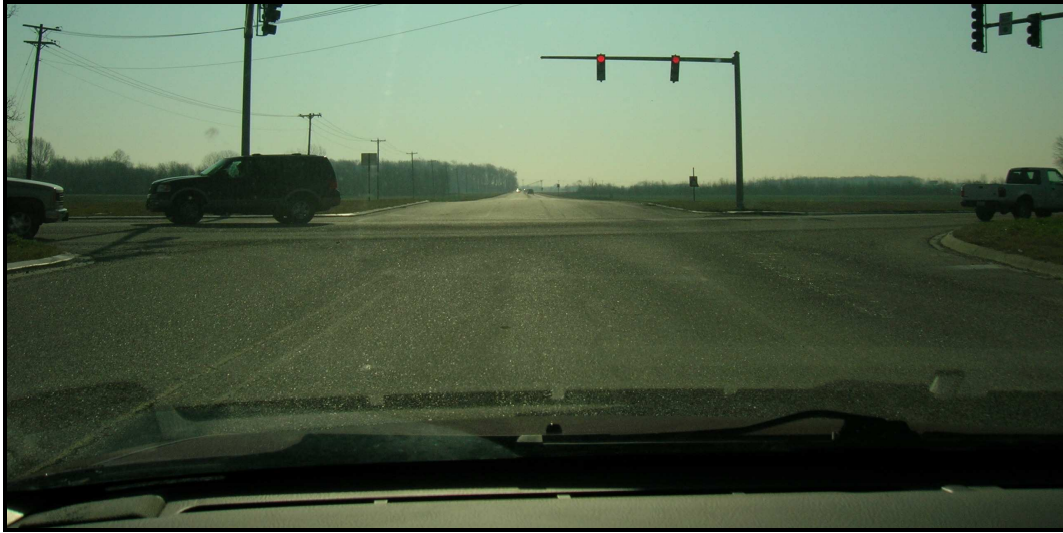
Figure 4: Worn Lane Markings (C1) – Location 17, Marion, Crittenden County
