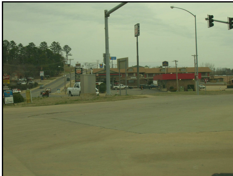
Figure 5: No Visible Lane Markings (C1) – Location 6, Clarksville, Johnson County
