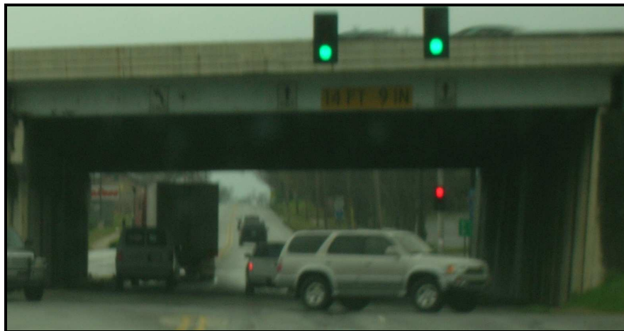
Figure 6: Poor Signage (C2) – Location 14, Little Rock, Pulaski County
