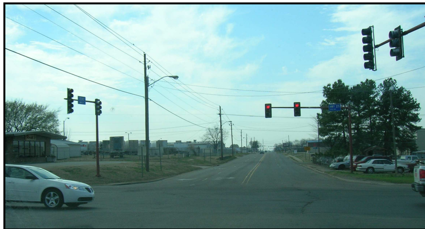
Figure 15: Traffic Signal on Corner (C6) – Location 12, Fort Smith, Crawford County
