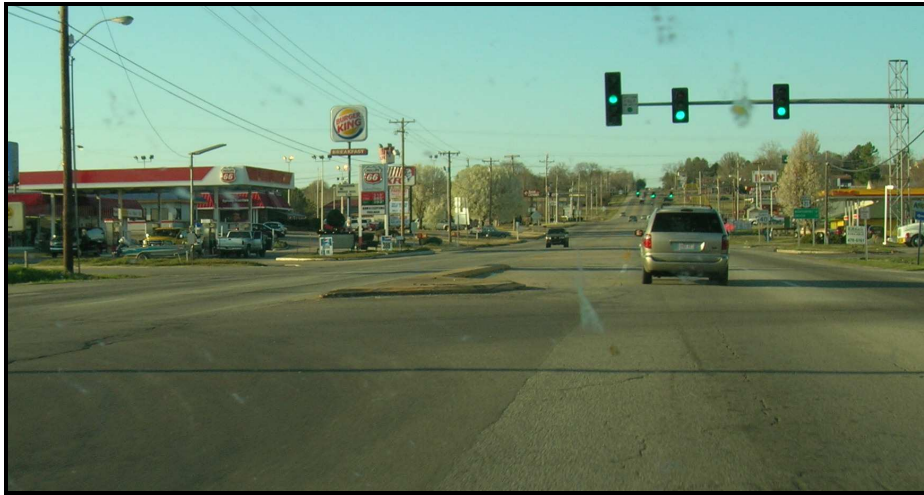
Figure 12: Median Before On Ramp (C5) – Location 1, Alma, Crawford County
